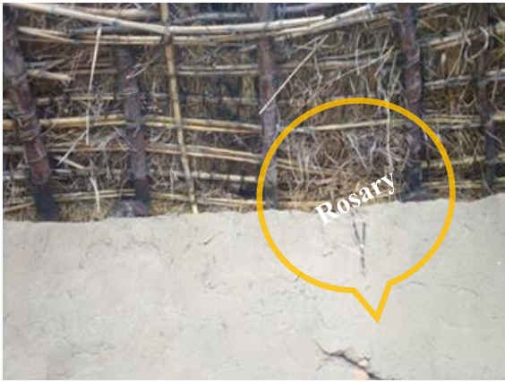
Fig. 4. Photo of the wall where thatch roof meets the mud wall. The inside was scorched by fire apparently started by lightning. A rosary was hung to chase away evil spirits.
