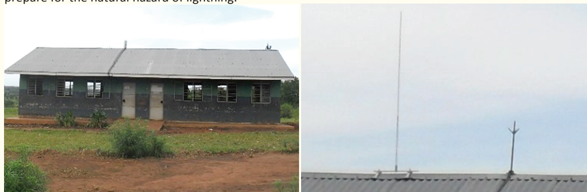
Left photo: Classroom building at Runyanya School where 18 children died and 38 hospitalized with lightning injuries in June 2011. Right photo: Close-up showing IEC compliant arrester installed by ACLENet and existing non-compliant multipronged rod commonly found on many Uganda schools that ACLENet staff have surveyed.
